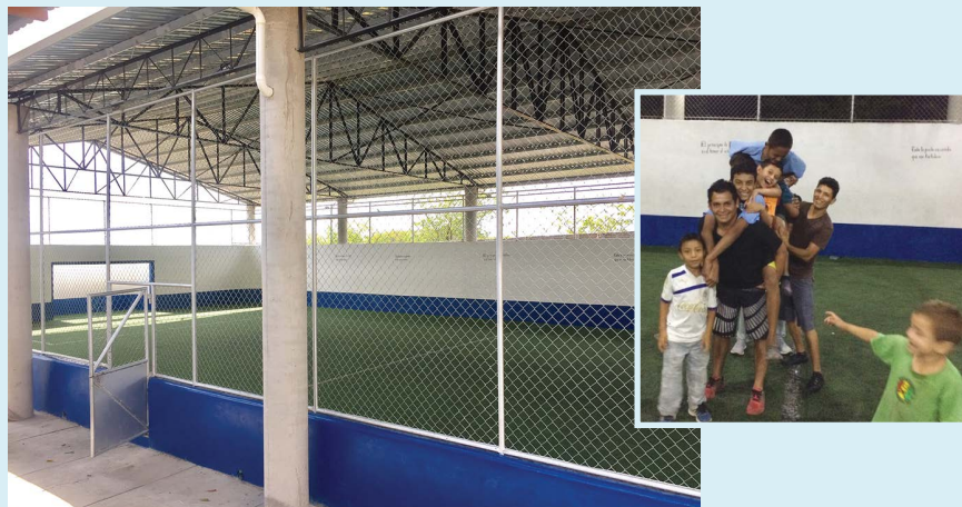
A new roof for the futbolito
