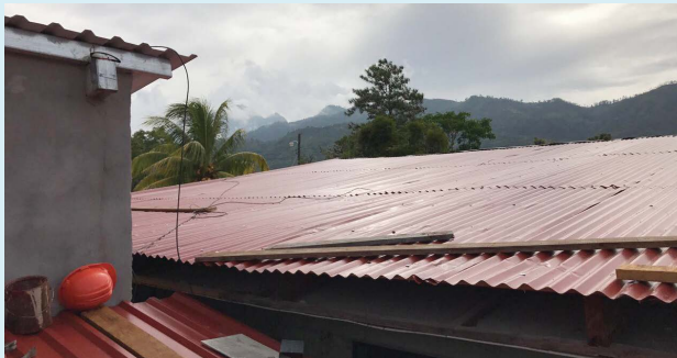
Roof repair in progress
